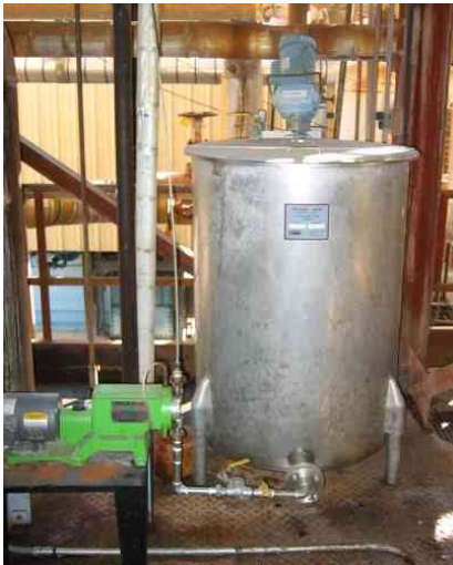
Citric Acid Addition System.. The Tank is SS 126 gallons and Chemineer top entering angle agitator, with a Pulsa metering pump series 880 diaphragm metering pump
